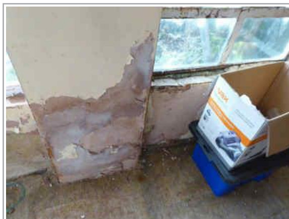
Damp issues and blown plaster
