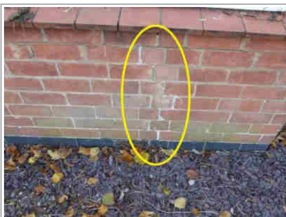
Cracking to bay window
