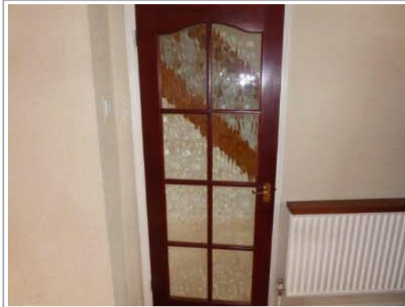
Probably non-dafety glazing to some internal doors
