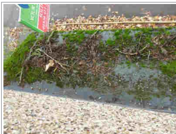
Felt roof covering to bay window from above
