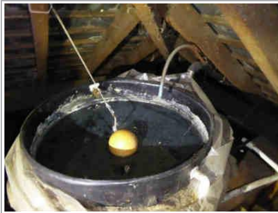
Uncovered and poorly lagged cold water tank in loft
