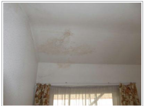
Water stained ceiling due to water penetration
