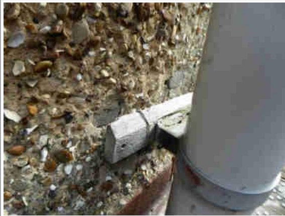
Re-attach fixing brackets to soil & vent pipe
