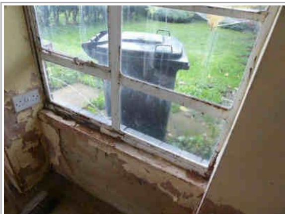
Low level and dangerous glazing
