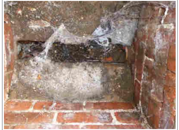
Partially blocked drain
