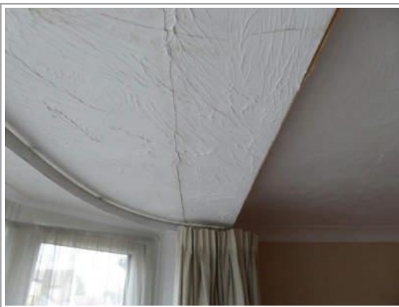
Bay window ceiling cracked and damaged
