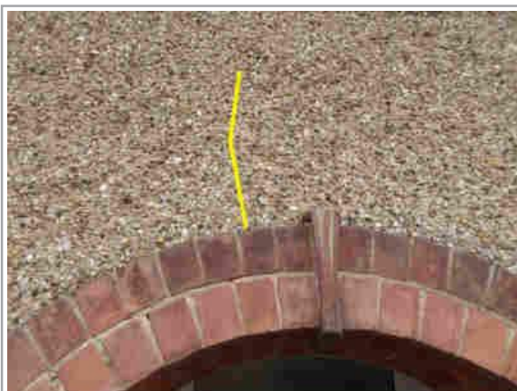
Minor render crack above porch
