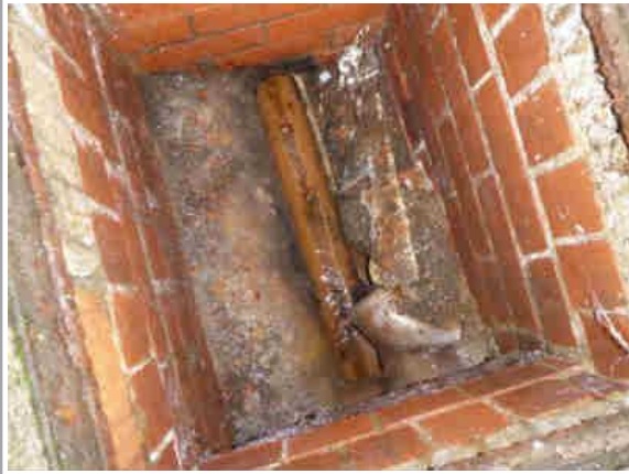
Minor repairs to haunching required
