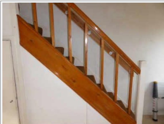
Spindle spacing a risk to children & handrail height too low
