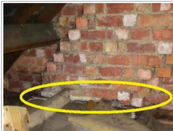
None standard support to flue above front bedroom
