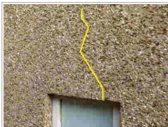
Cracking to right gable
