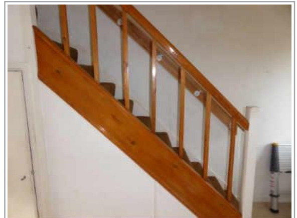
Spindle spacing a risk to children & handrail height too low
