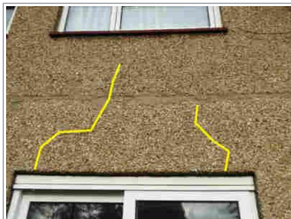
Render cracking to rear
