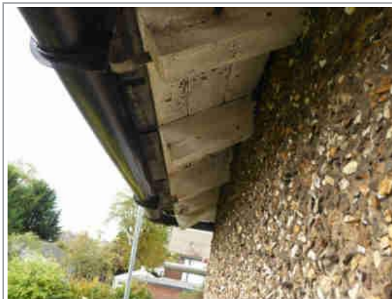
Redecorate rafter feet & soffits as normal maintenance
