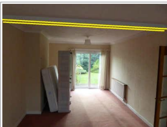
Wall removed between the two reception rooms
