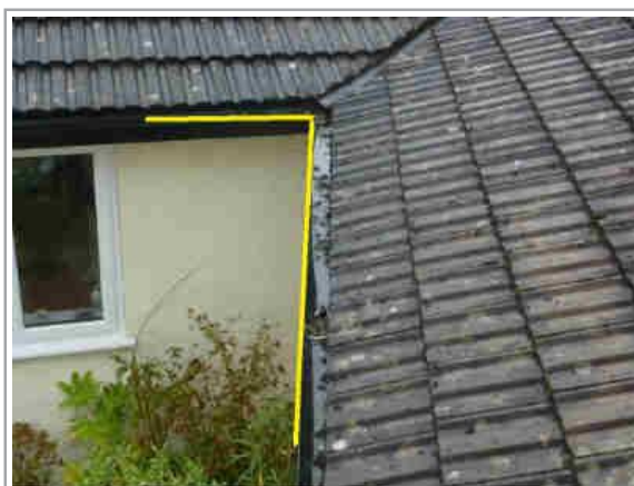
Clean realign and reseal gutters
