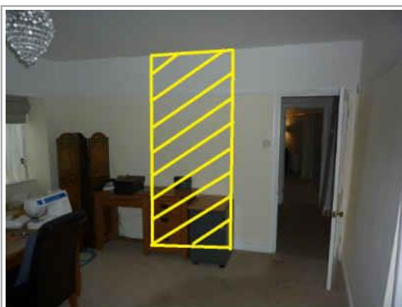
Site of removed chimney breast in dining room
