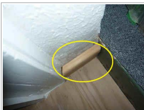
Small section of skirting requires fixing to wall
