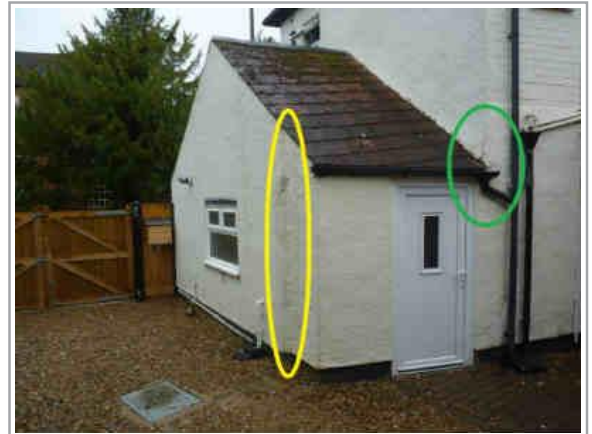
Limited verge detail leading to rainwater draining down the gable end
