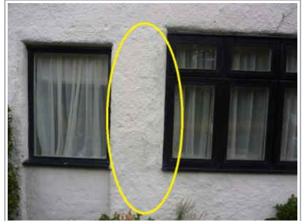
Repair to render required
