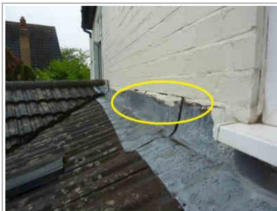
Minor re-bedding of lead flashing required
