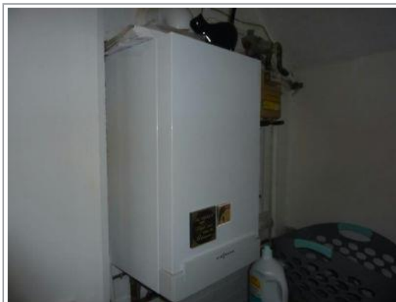
Gas boiler in utility room
