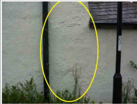
Blown render to the front elevation
