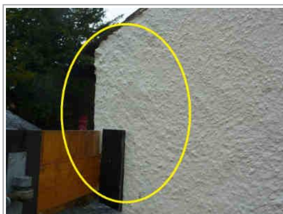
Hollow render to right of utility wall
