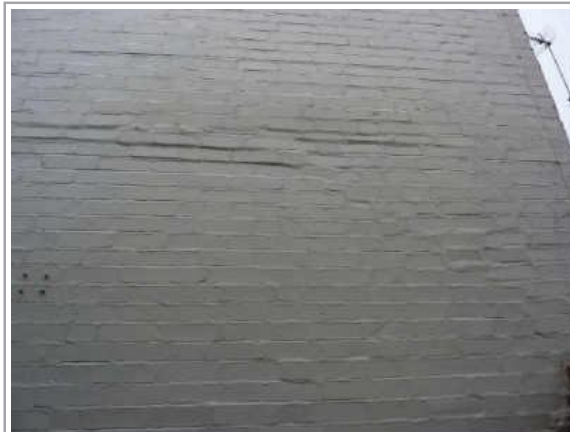
Repointed and painted brickwork masks previous alterations/movement and workmanship quality
