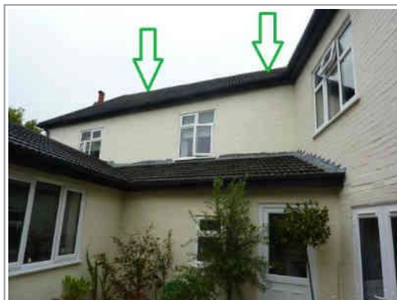
Moderate deflection to roof timbers due to heavier roof covering
