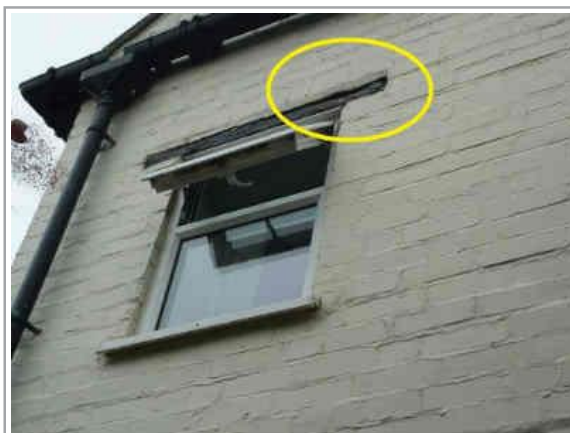
Minor repair and redecoration of bedroom window lintel required
